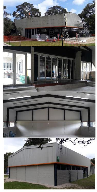
automated roller shutters to enclose the space and the existing skylights were upgraded to be BAL29 compliant. The PAC extension and enclosure was designed and built to BAL29 (Bushfire Attack Level) and complies with relevant design codes.
