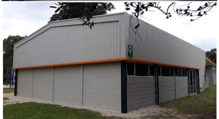
automated roller shutters to enclose the space and the existing skylights were upgraded to be BAL29 compliant. The PAC extension and enclosure was designed and built to BAL29 (Bushfire Attack Level) and complies with relevant design codes.
